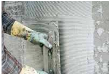
Hand applied mortar
