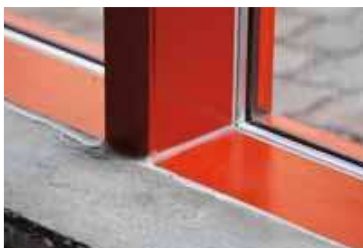
Sealing of connection joints around windows and doors
