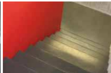
Flooring for vomitories and stairways
