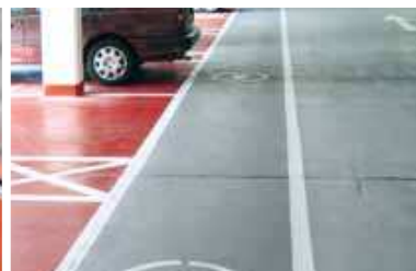
Sealing of floor joints in carparks and elsewhere
