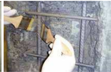
Protection of steel reinforcement
