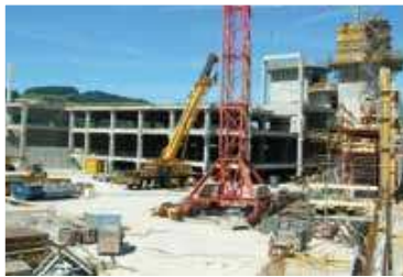
Site batched concrete production
