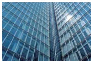
Sealing of glass façades
