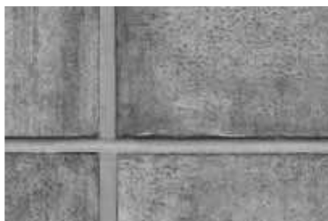
Sealing of stone, brick and concrete joints
