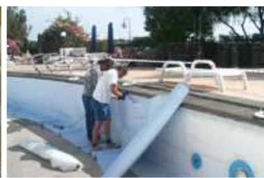
Waterproofing with flexible Sikaplan
