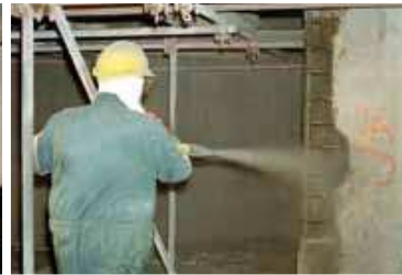
Machine applied concrete repairs
